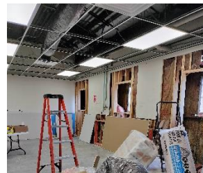
Drywall and drop ceiling progress
