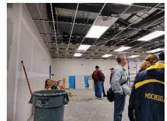
Drywall and drop ceiling progress
